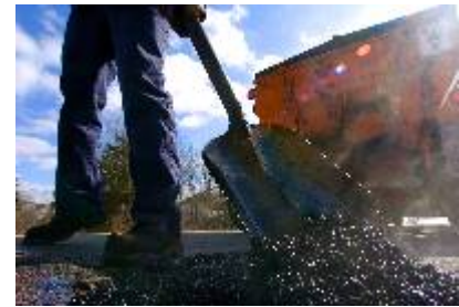
West Side streets division worker Terry Richardson scoops filler into a pothole Wednesday along South High Point Road, near Velvet Leaf Drive. (Photo by John Maniaci - State Journal)
